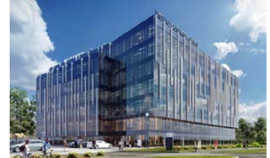
Vistula Business Garden Kraków (Poland)
